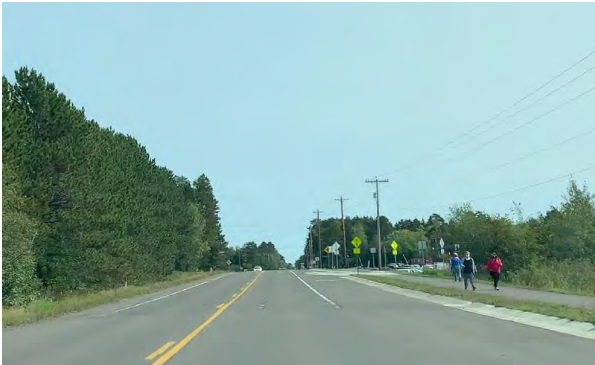
Big Lake Road looking east (west of Trettel Lane) Source: Associated Consulting Services, 2020
